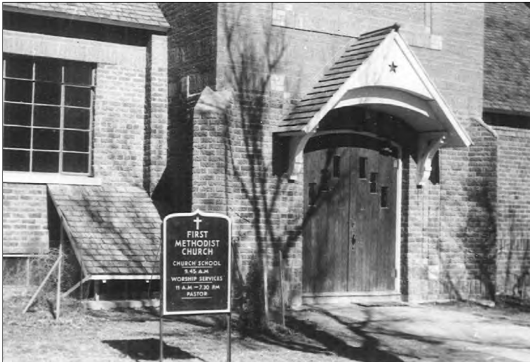
Figure 5. This April 1958 image (view northeast) provides a detailed view of the church entrance. Courtesy First United Methodist Church, Eads, Colorado.
