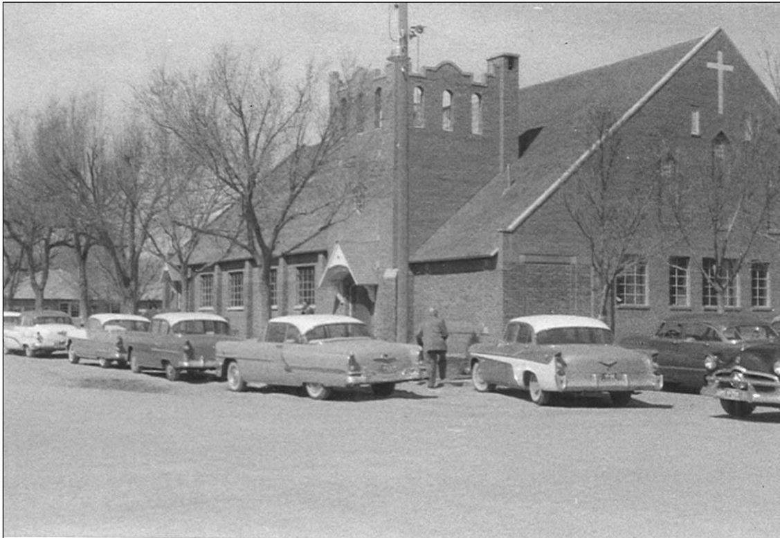
Figure 3. The congregation finally completed the church in 1951. The south (left) and east walls of the finished church are shown in this April 1959 view (northwest). Courtesy First United Methodist Church, Eads, Colorado.
