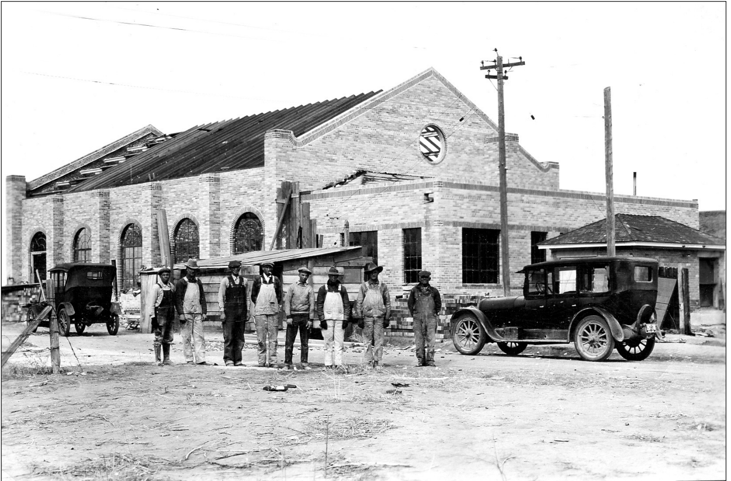
Figure 1. Workmen pose in front of the unfinished gymnasium in this ca. 1929 view northwest. Courtesy of Eads High School, photograph collection, undated.
