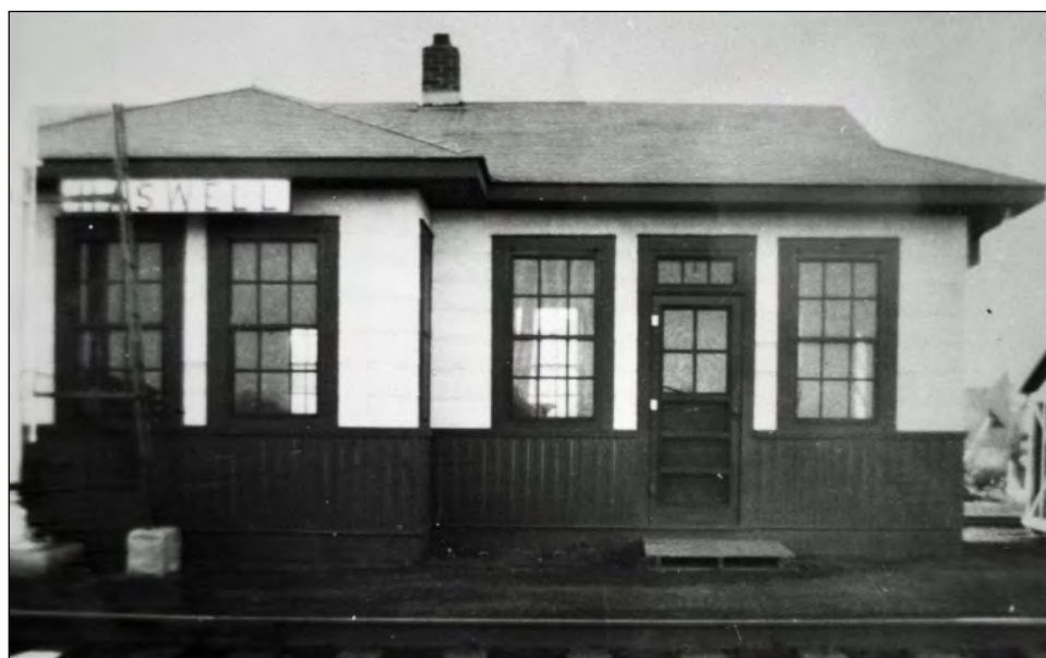
Figure 2. The smaller ca. 1950 replacement frame depot featured walls clad with asbestos cement shingles and vertical beadboard. Courtesy of Kiowa County Public Library, Railroad Collection, date unknown.
